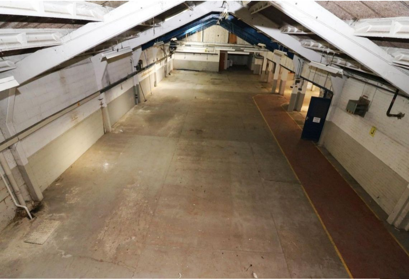
LON4296 London Warehouse Gritty Interior For Filming
